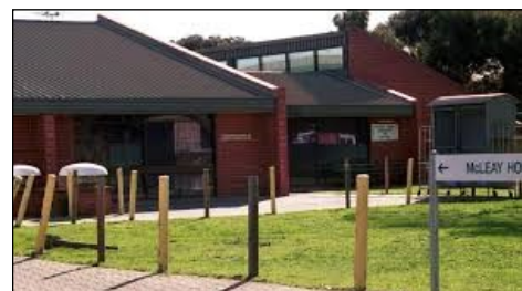
Makk and McLeay Nursing Home is part of the Oakden complex
